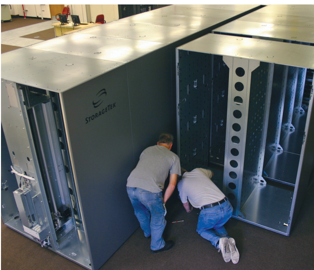
Figure 4 Construction of the Sun SL8500 ATLs.
